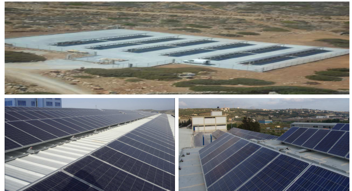
Pictures 4, 5 and 6: Views of Plastika Kritis photovoltaic stations nearby the Wind Farm (top) and at the roofs of its plants in Iraklion (bottom left and right)
